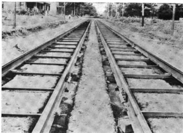
CONCRETE GIRDER CONSTRUCTION IN COLUMBUS READY FOR CONCRETE
