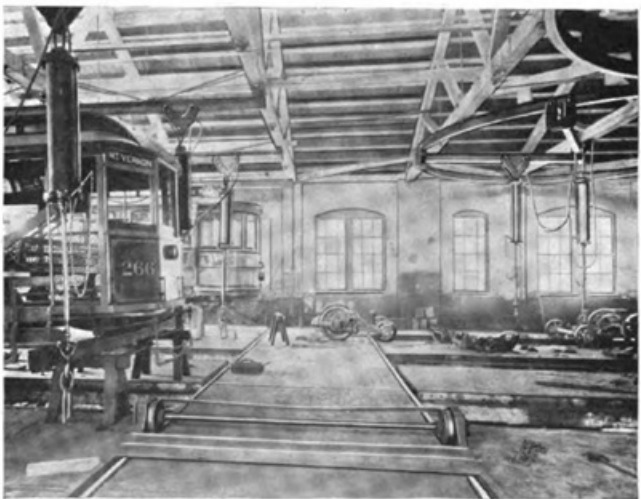
CAR SHOP, SHOWING CIRCULAR CRANES AND TRANSFER TABLE
