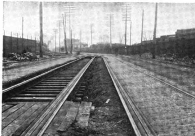
DOUBLE-GAGE TRACK IN COLUMBUS
